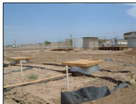
Lined trenches after planting
