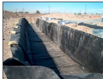
Lining the Trenches
